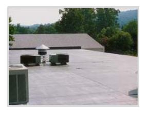
**OVER 40 YEARS OF FIELD PROVEN PERFORMANCE.** One of the first EPDM roofs was installed in 1965. That roof is made with our Royal Edge polymer, and is still in service today.
